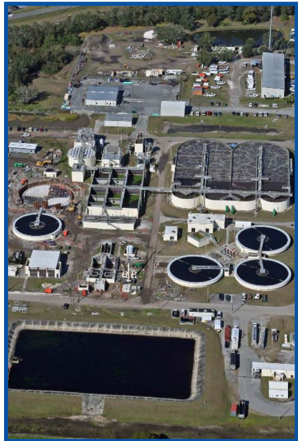
South Bermuda Water Reclamation Facility
