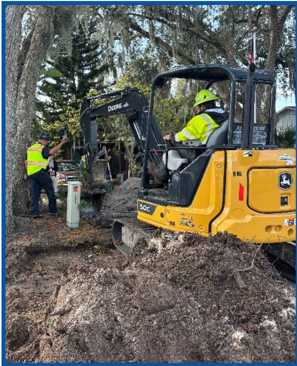
Sewer Lateral Installation
