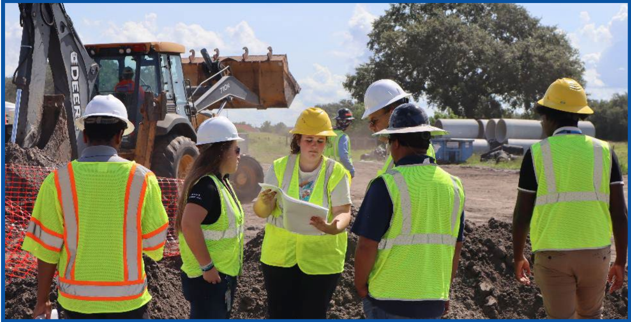
Engineering oversees Horizontal Directional Drilling Project
